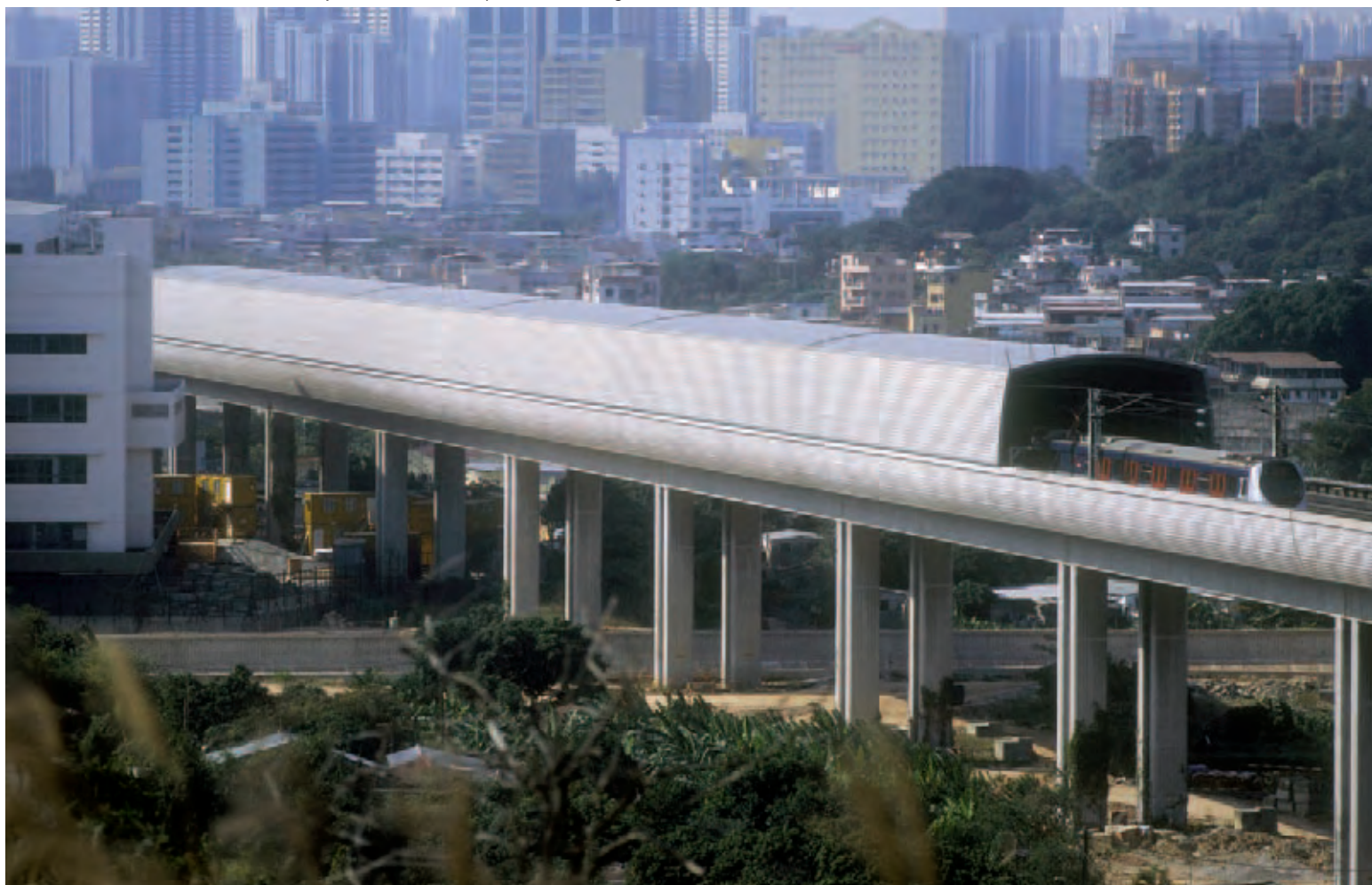
11. The full noise enclosure in use, adjacent to Pok Oi Hospital at Yuen Long.
