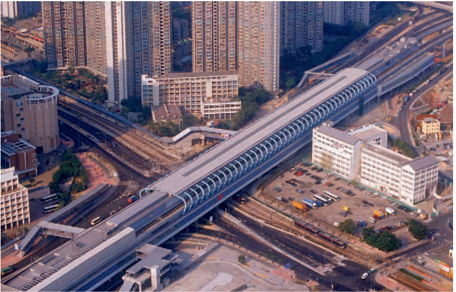
21. Roof cladding at Tin Shui Wai station.
