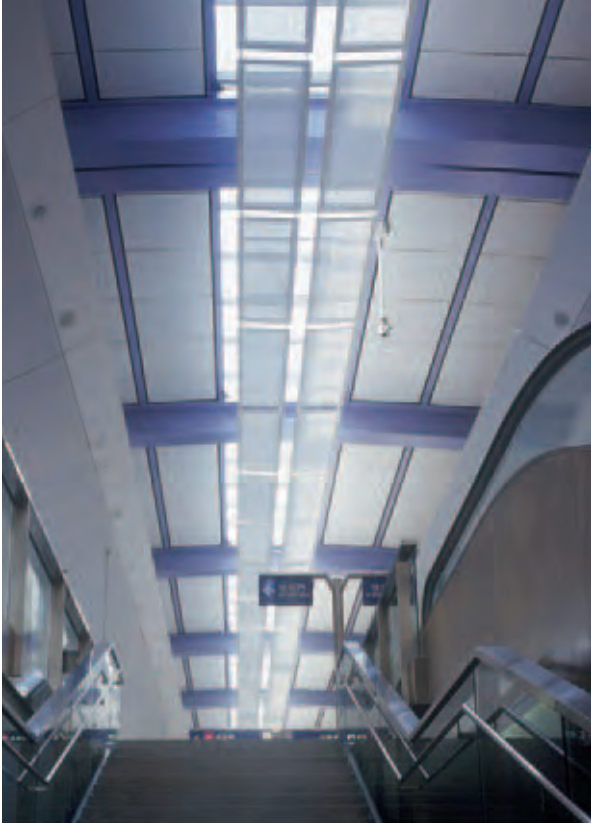
18. Central rooflight at Tin Shui Wai station.
