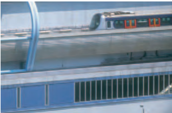
19. Full-height "slit" windows at Tin Shui Wai station.
